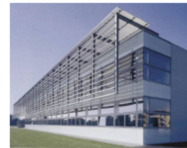
View of longitudinal facade with sun protection
