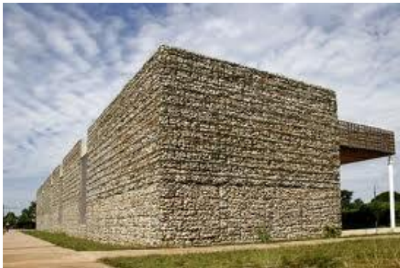
Walls from local stones
