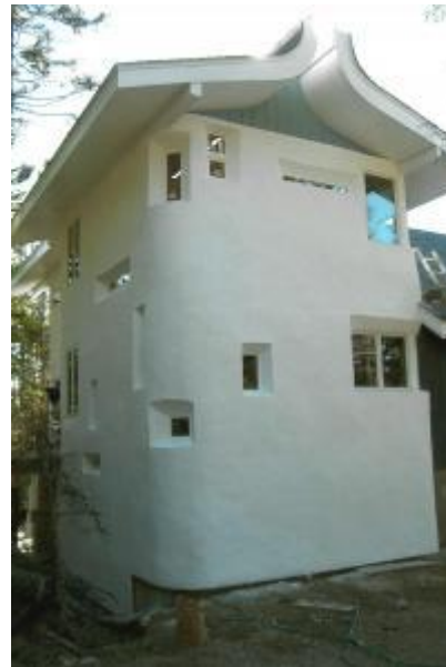
Biological insulation materials applied
